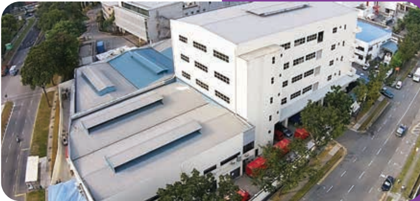
■ Our modern food manufacturing facilities at 30 Senoko South Road Singapore 758088
